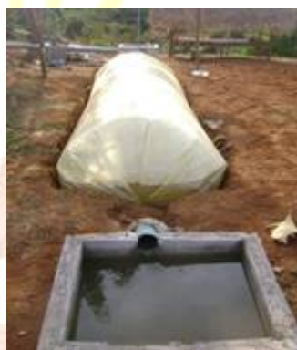
Figure. 3. The plug-flow tubular polyethylene biodigester
